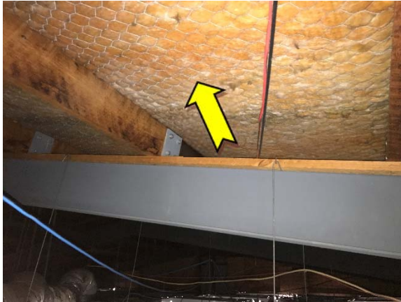
Photo 7. Interior, level 1, throughout ceiling space – suspected SMF sarking insulation.
