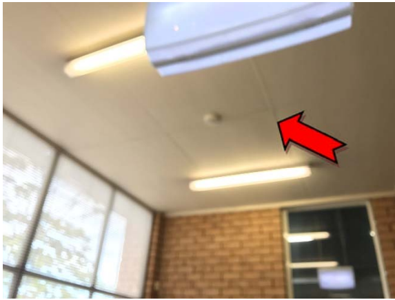
Photo 3. Interior, ground level, office area, ceiling – asbestos-containing fibre cement sheeting.
