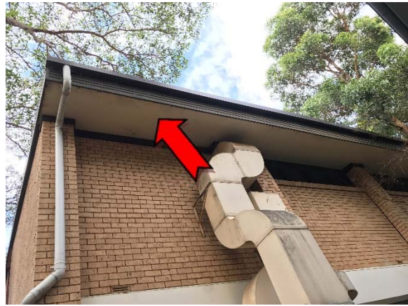
Photo 4. Exterior, north and south elevations, eaves – asbestos-containing fibre cement sheeting.
