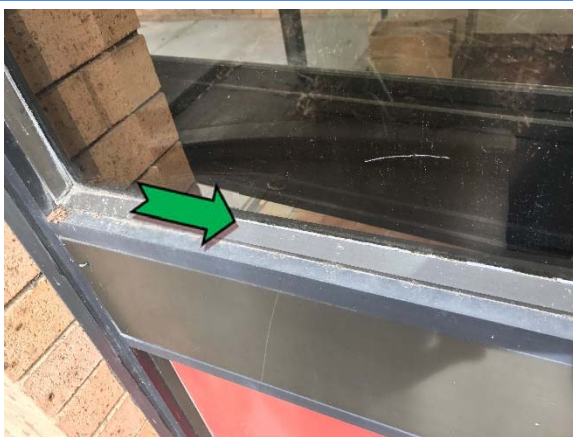
Photo 5. Exterior, throughout, window frames – non asbestos-containing window caulking.
