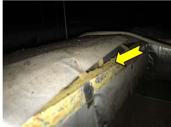
Photo 8. Interior, level 1, throughout, ductwork – suspected SMF internal insulation.
